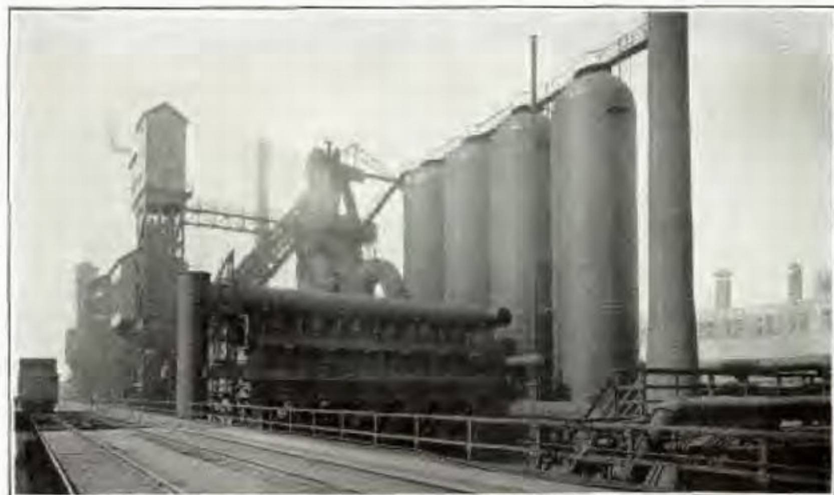
A Fine View of One of the Blast Furnaces as Seen from the High Line.
