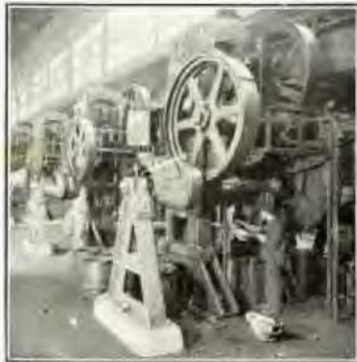
Huge Presses for Forming the Crankcase
