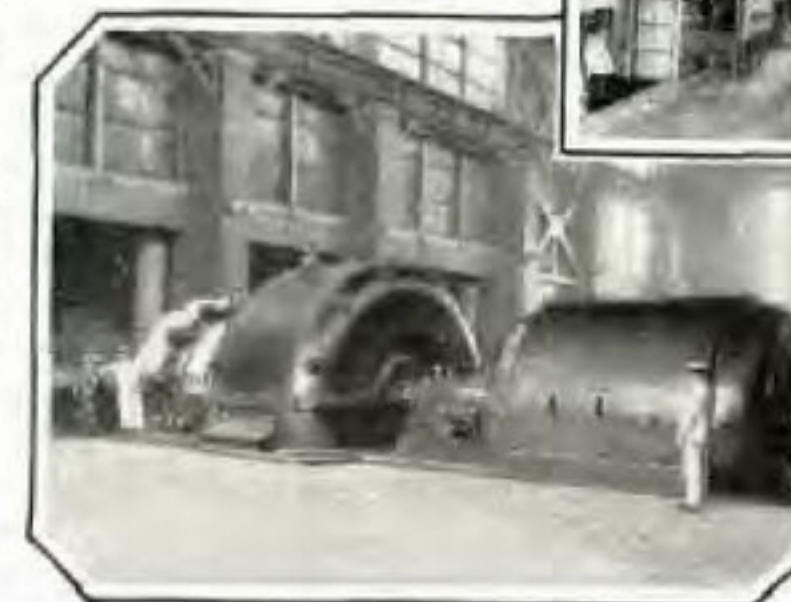
The Furnace Room. Left: 62,500 H. P. Turbo Generator
