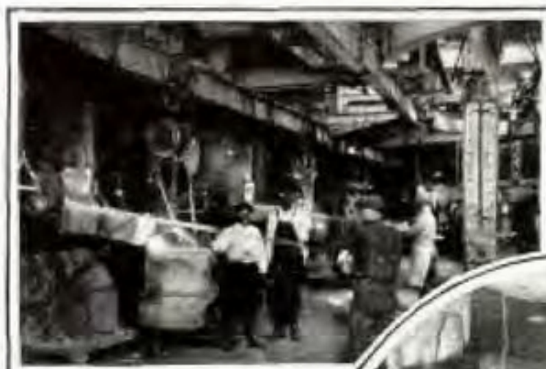
Filling a Ladle at a Cupola.
