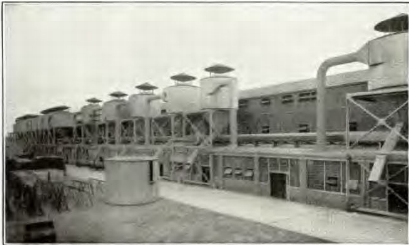
A Building Where Wood Working is Carried On.—Note the Dust Collectors to Keep the Air Clean.
