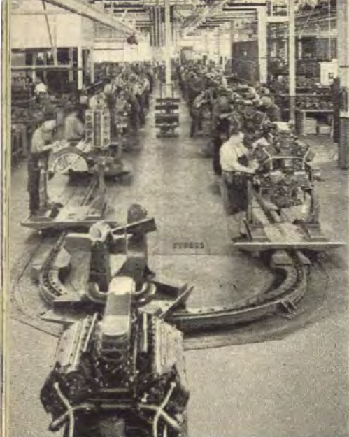
Here in light, clean and airy surroundings the Ford V-8 Tank Engine is assembled. This is typical of Ford working conditions.
