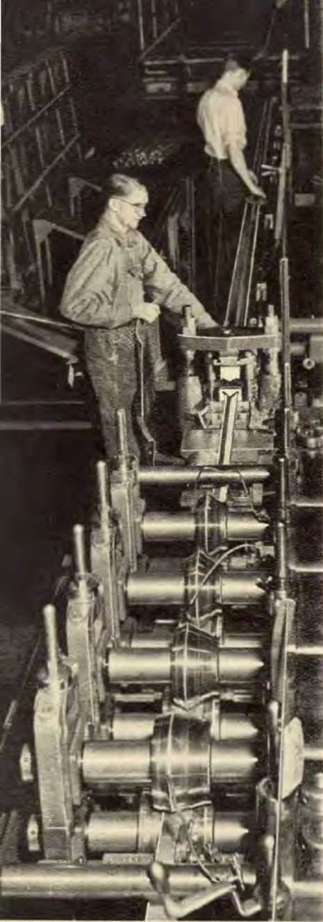
A Liberator began here. This former shapes aluminum strip into channel beams and ribs. Later, these are stretched to size, making them stronger.
