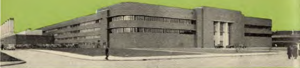
A $27,000,000 air conditioned building was constructed in record time in spite of winter weather. The entire structure was housed in a weatherproof "cocoon" so that work could proceed. Ground breaking ceremonies were held September 17, 1940, and the building was completed and ready for use March 17, 1941.
