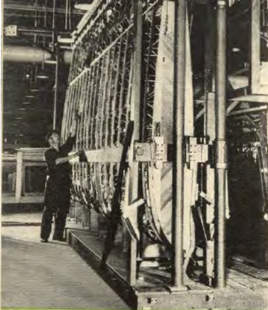
Complex wing structure of the CG-4A is shown by this scene on the production line at Iron Mountain. Interior bracings were glued by a special patented Ford process.
