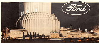
A reception to Hugh Ferriss, noted New York artist, of how the Ford Exposition Building appears at night in its maze of flood lights. The structure is 900 feet long and equivalent to 13 stories high in its central section. It faces upon a five-acre park fronting on Lake Michigan.
