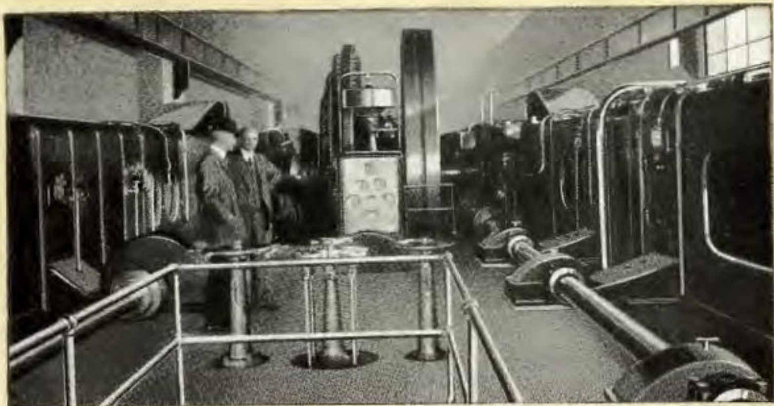
6,000 h. p. Engine—Showing Starting Devices
