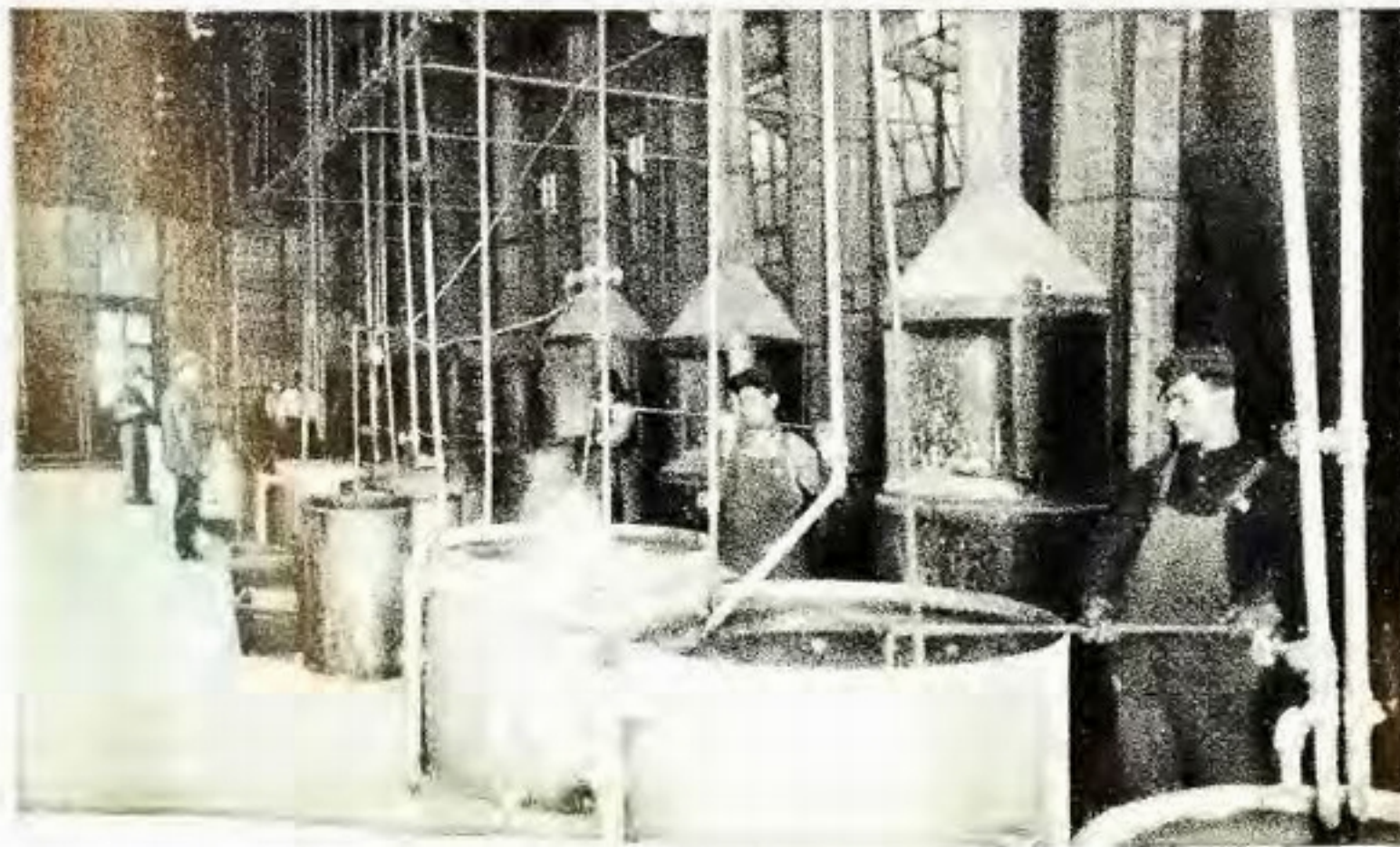
Cyanide Pots and Quenching Tanks
