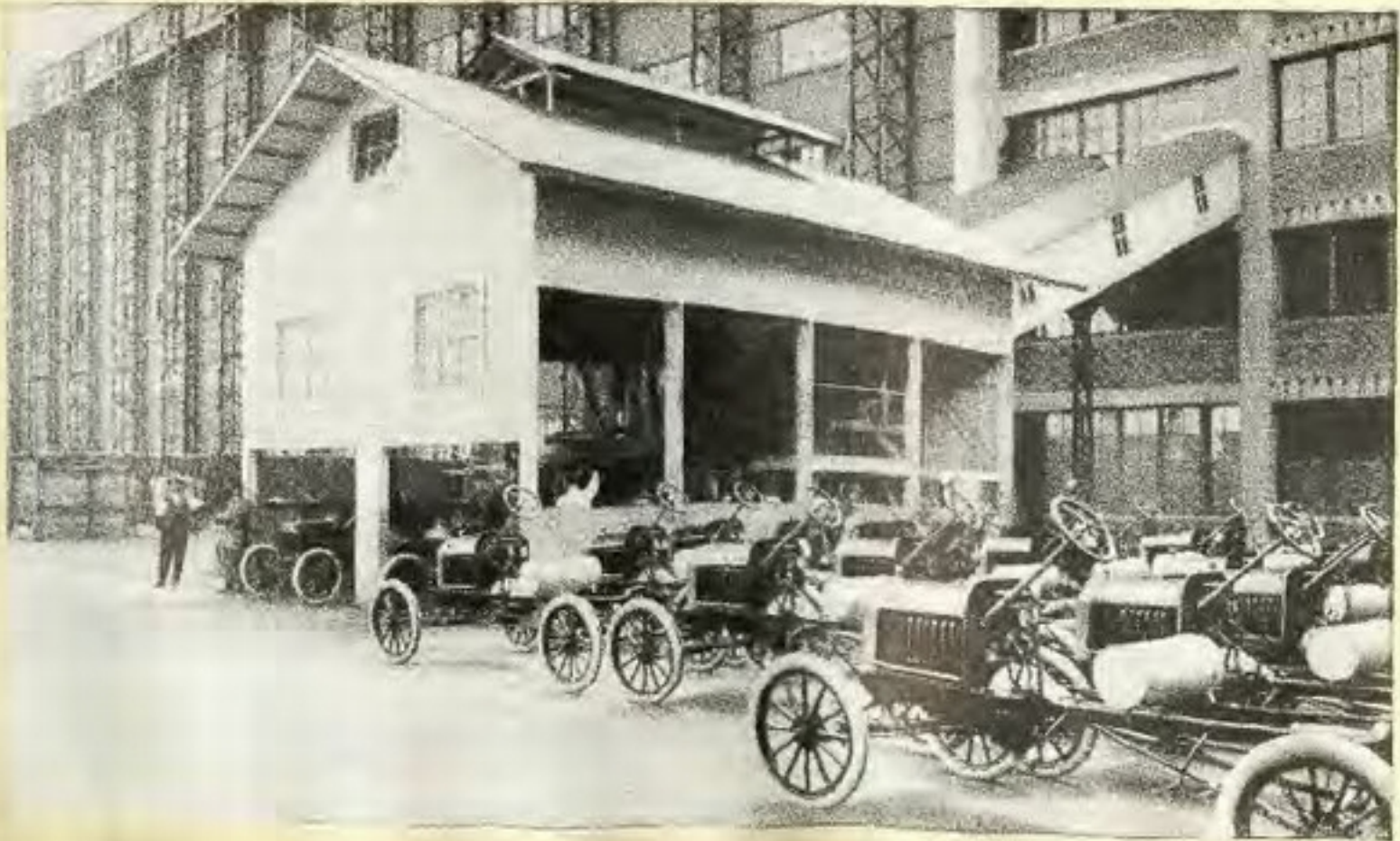
Part of New Six-Story Building—Showing the Body Chute
