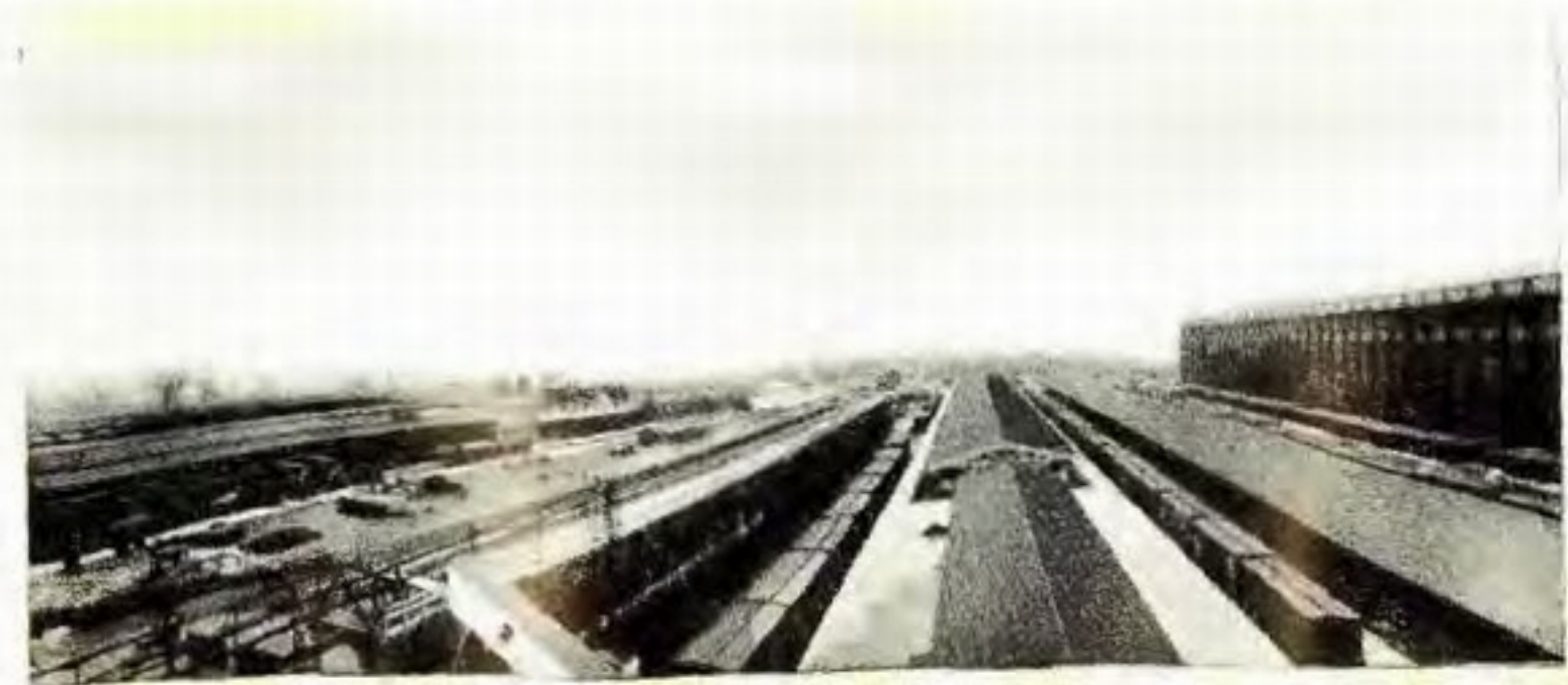
General View Factory Yard
