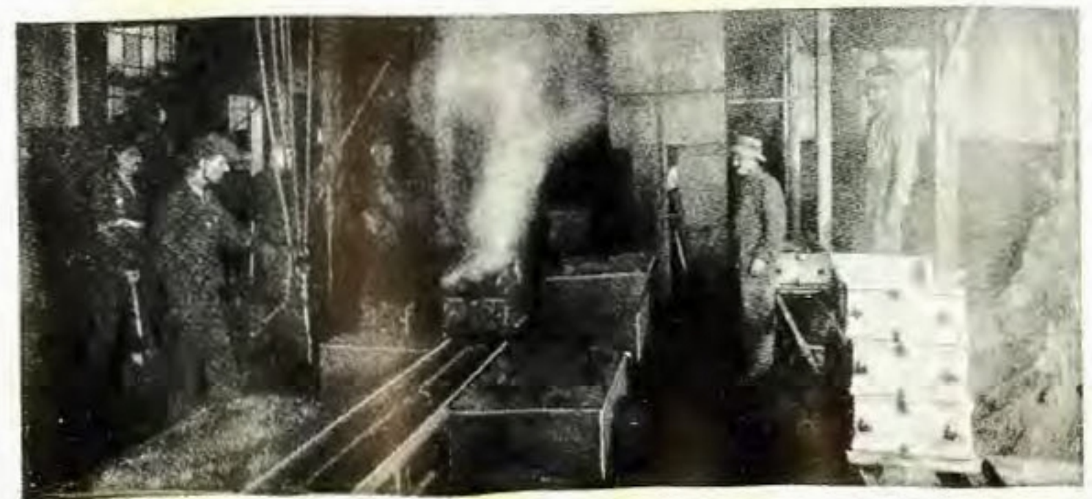
Breaking the Cylinder Moulds
