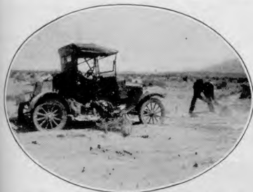
Effecting a Temporary Improvement in the Road Bed
