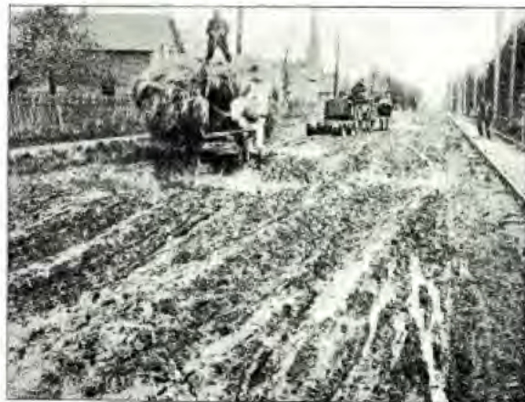
Gratiot Road out of Detroit, before improvement
