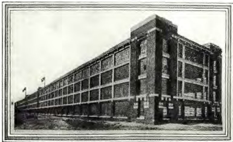
Part of the new Ford Plant
