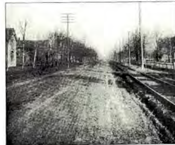
Gratiot Road after improvement
