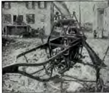
The above photographs show the latest achievement of one of our Boston owners. This machine actually flew—made several successful flights. Notice how the builder cut the radiator in two and used a half an each side
