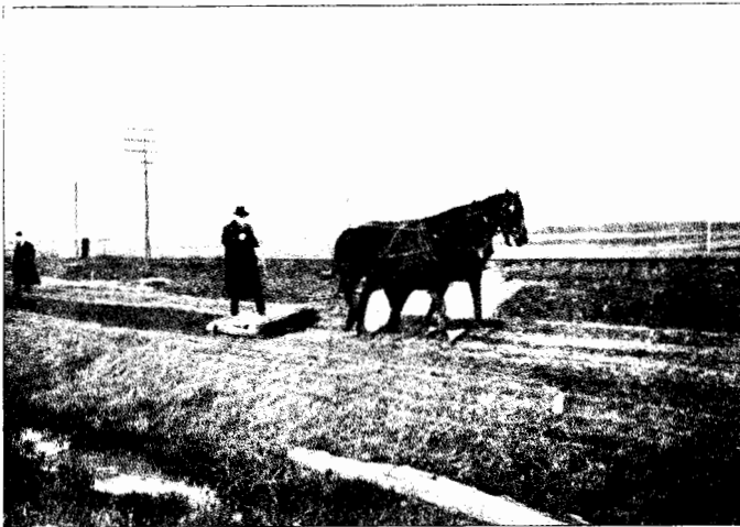
The Log Drag in use on a muddy road. The two horsepower team as shown in the picture is fast losing its popularity and the automobile is taking its place
