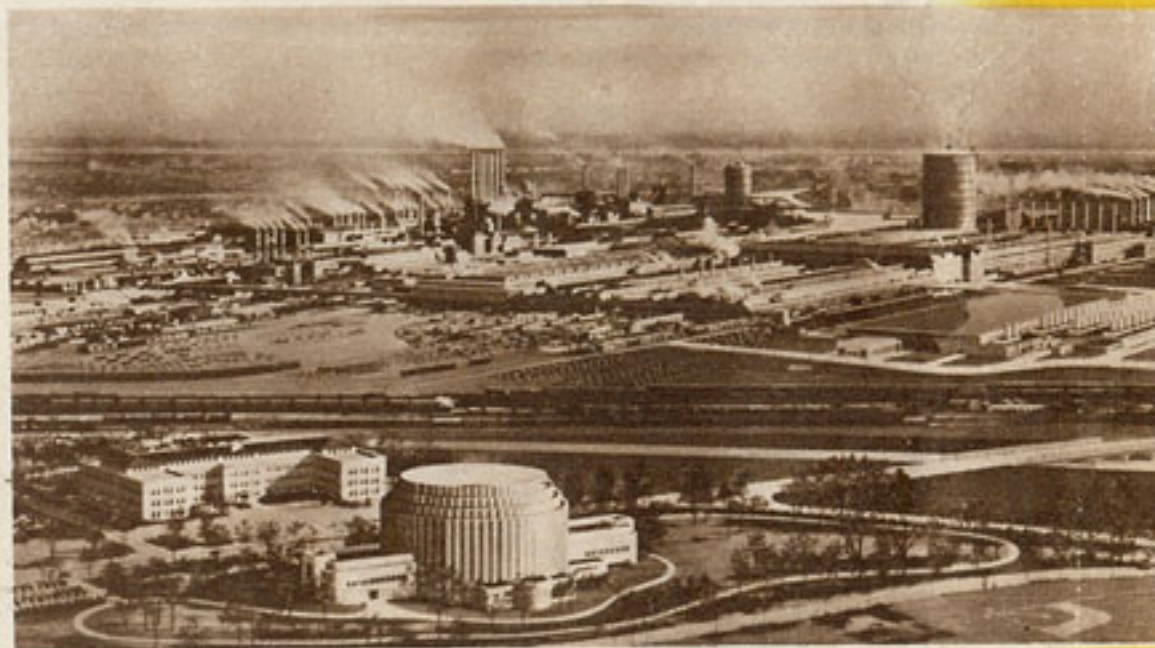
Manufacturing Metropolis. Today the great Rouge Plant, hub of Ford production activities, covers more than 1,190 acres with docks, railroad, bus line, blast furnaces, coke ovens, steel rolling mills, glass plants and numerous shops and assembly lines.
