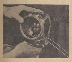
With synchronizing completed, the Lincoln-Zephyr coil, if checked and found acceptable, may now be altered to fit new distributor assembly. Remove brass springs with a pair of diagonals. These springs were originally the source of voltage for the stock Lincoln-Zephyr points. After removing springs, cover with rubber cement and place a piece of electrical rubber type tape over cavities.
